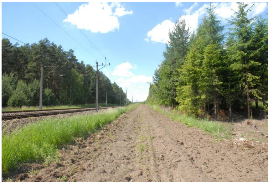
Figure 2. Modified firebreak beside the railway
