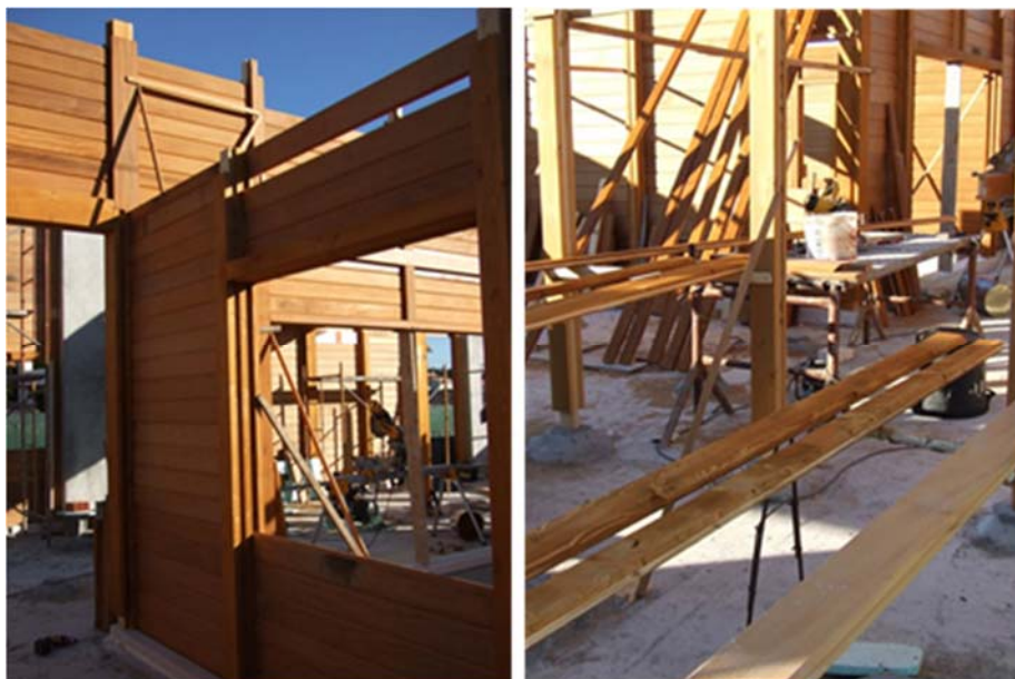
Figure 1. Wood-framed house under construction
