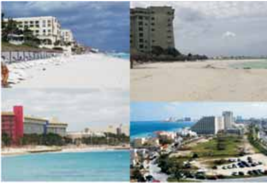
Fig. 26: other views of the built environment that is typical of the hotel resort area in Cancun. The views on the left of this figure show several hotels built on the water side of the dune of the original island and the use of retention walls to allow for landscaping and even sand to be maintained on the waterfront of these buildings. The pictures on the right show buildings on the northern man-made land bridge linking the original Cancun Island to the mainland, which has no dune allowing for buildings to be built even closer to the waterline and at lower elevations (as low as only 1.5 to 2 m above mean sea level) with respect to mean sea level.
