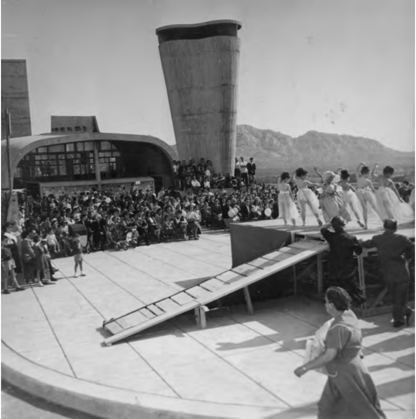
27. Unité d'Habitation in Marseilles. Roof terrace during inauguration ceremony on October 14th, 1952. Unknown photographer.
