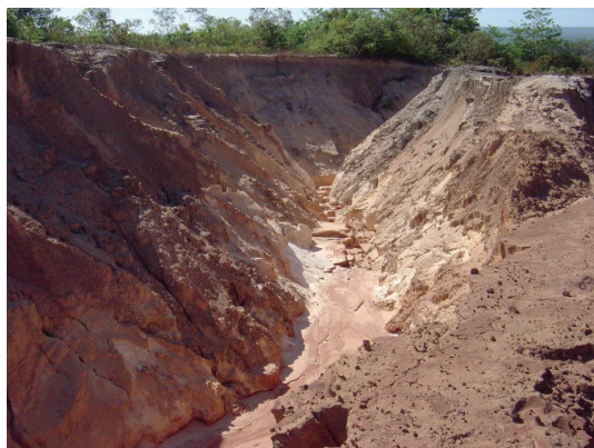
Figure 1 The lithological conditions of Serra do Cachimbo, on the border of the states of Mato Grosso and Pará, did not resist, and after 5 years of the construction of BR-163, it presents gullies of great dimensions that make the road traffic difficult. Currently, this stretch is paved with asphalt.
