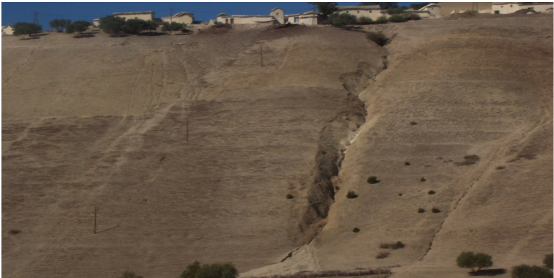
Figure 8 Deeply incised gully formed on the steep slope in Leben Watershed in Prerif area. The situation of September 2015.
